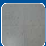
VCT (Vinyl) tile and linoleum
